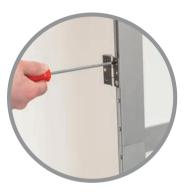
Slide one side of first hinge with connector bar into same channel of post in which the door threshold is secured. Slide second hinge into channel of vertical profile, on opposite side to lock and handle, until it rests on connector bar in the door. Tighten two screws to secure hinge to door frame.
